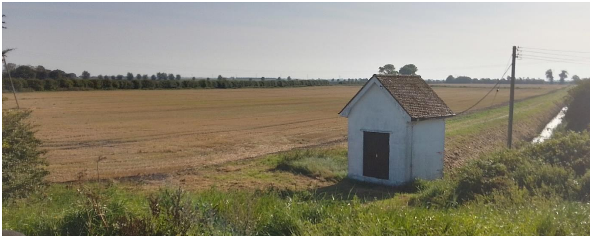
Ouse Bridge farm drainage pump. The field earmarked for rewetting are behind the pump and disappearing into the distance on the right.
